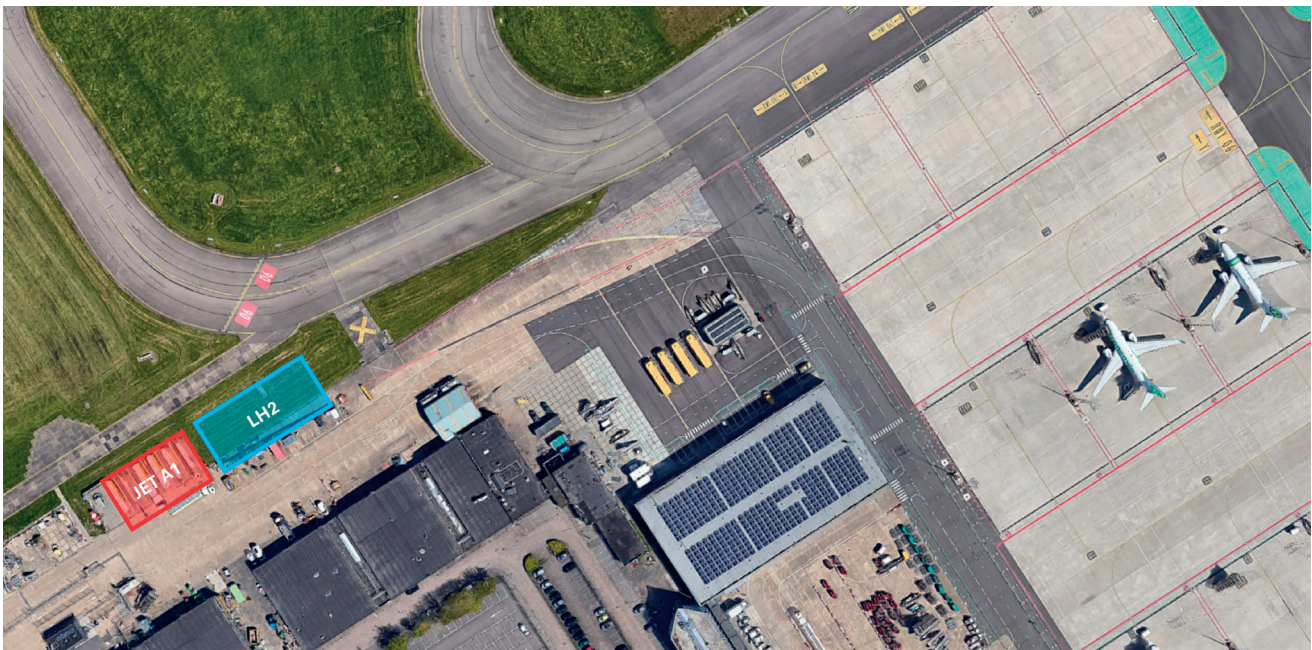
Figure 16 Current JET-A1 mobile storage facility at RTHA and a size comparison for a LH 2 mobile storage facility that accommodates 12 trailers (the exact location and details of the infrastructure are subject to the outcomes of the GOLIAT project and future developments in the specific domain of airport hydrogen infrastructure)
